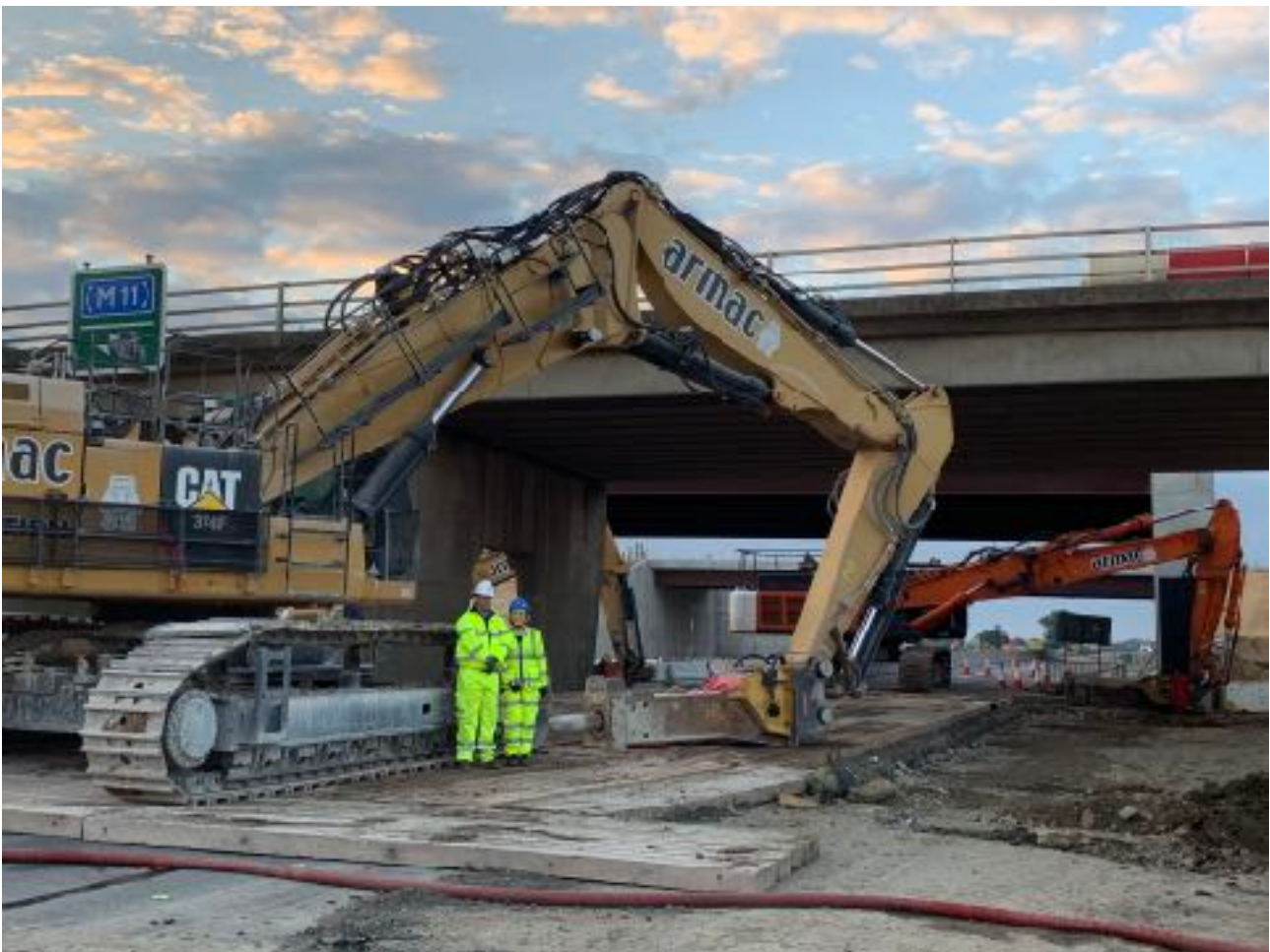
Photo taken at about 5am just before the demolition started.
